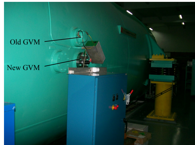
Figure. 4. The two generating voltmeters installed on two neighbor ports of the tandem tank.
